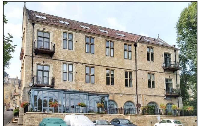
The apartment building from the east.
