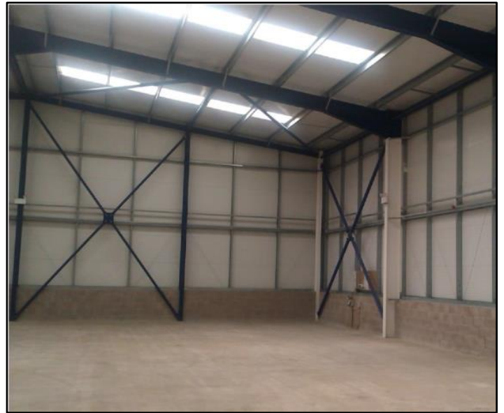
Interior before fit out.
